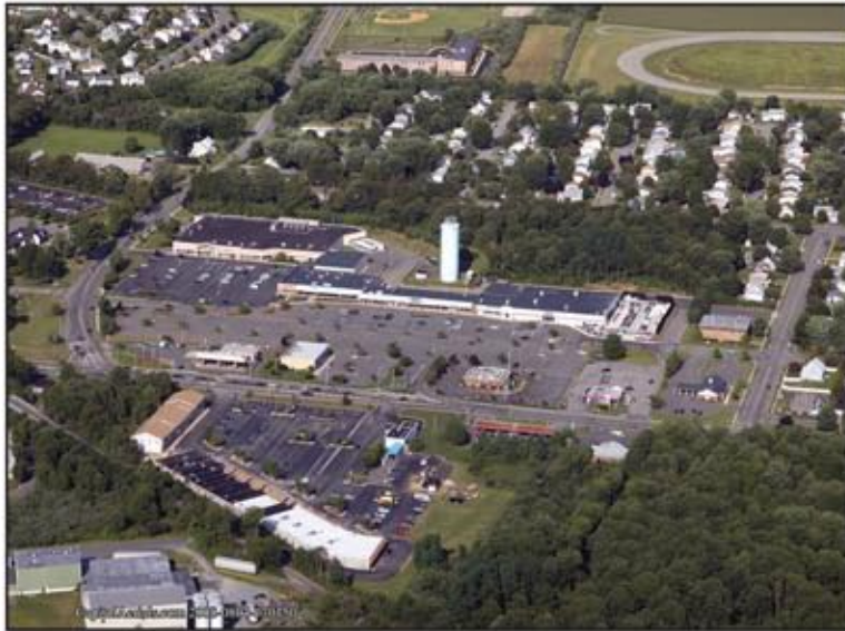
Sutton Plaza on Rte. 206 in Flanders aerial
